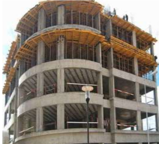
Fig 1: Conventional Slab
