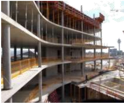
Fig 2: Flat Slab
