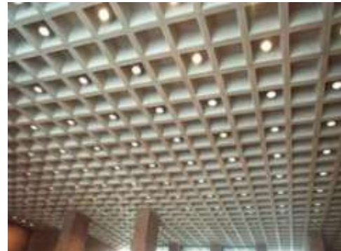
Fig 3: Waffle Slab
