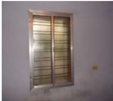
Fig 2.1 – Installation of window
