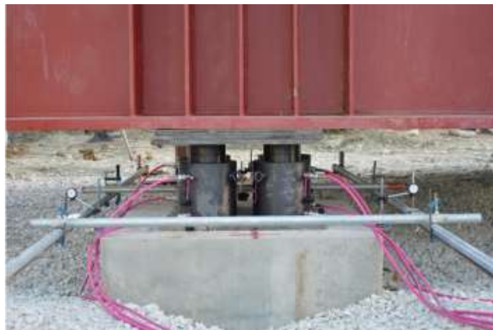
Figure 9. Installation of 4 hydraulic jacks on the bridge 3, piles nr 3
