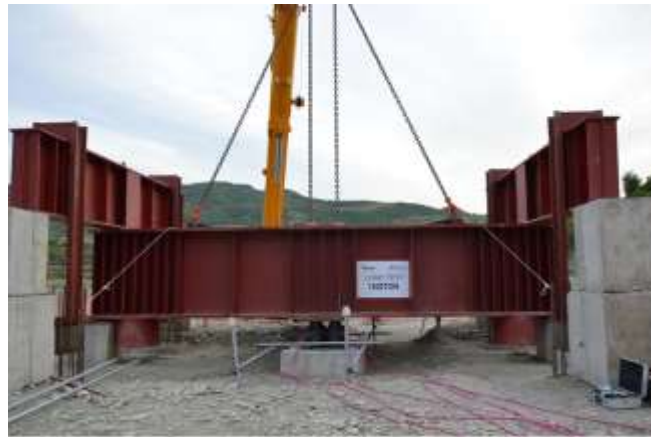
Figure 8. General layout installation of steel frame during load test on the bridge 3, piles nr 3
